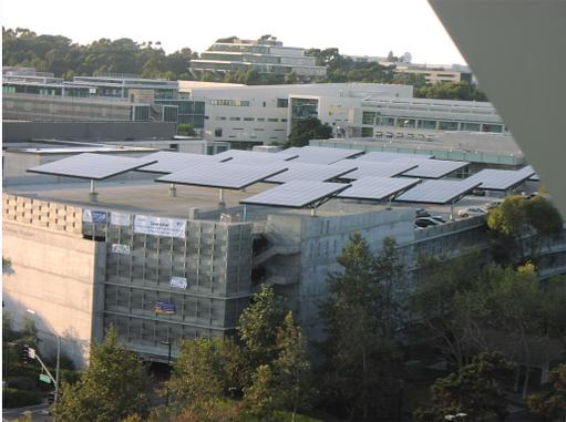
At present, UCSD has installed 1 MW of solar PV, online since Dec. 2008. UCSD uses 30 MW, 25 MW generated on campus (gas turbines, mainly)
