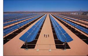
**Solar Thermal:** ~30% efficient; cost-competitive; requires direct sun; heats fluid in pipes that then boils water to drive steam turbine
