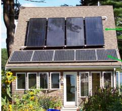
**Solar hot water:** up to 50% efficient; several \$k to install; usually keep conventional backup; freeze protection vital (even in S.D.!!)
