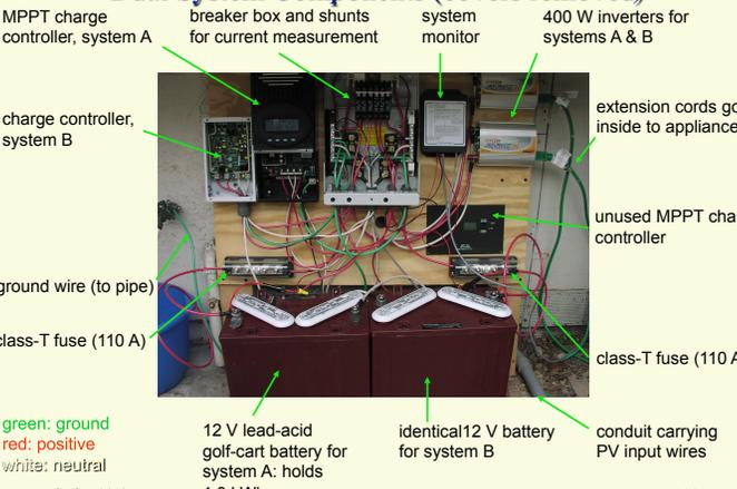
MPPT charge controller, system A    breaker box and shunts for current measurement    system monitor    400 W inverters for systems A & B
